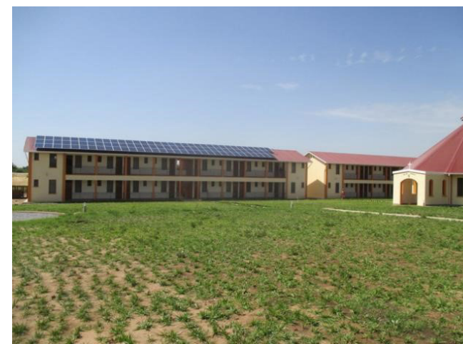
The Good Shepherd Peace Centre, South Sudan supported by Shalom-SCRR with fully accessorized Solar Lighting System - enough to power the whole institution.
