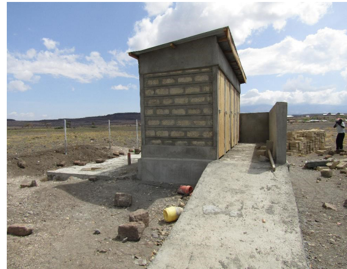
Construction of standard latrines/toilets: Good latrine conditions at school have improved the school environment by meeting specific health and hygiene/sanitation needs of both boys and girls and to a significant extent reducing absenteeism .
