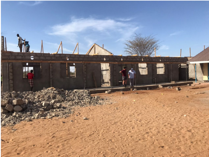
Shalom-SCCRR's Executive Director, Fr. Oliver Noonan MA (PhD. Candidate) and Mr. Ciaran King, witnessing an ongoing construction of classrooms funded by Shalom-SCCRR in Turkana County, Kenya.
