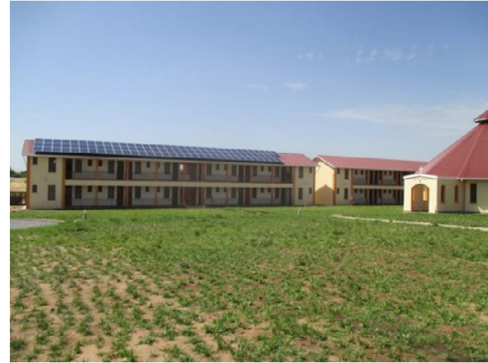
The Good Shepherd Peace Centre, South Sudan supported by Shalom-SCCRR with fully accessorized Solar Lighting System - enough to power the whole institution.
