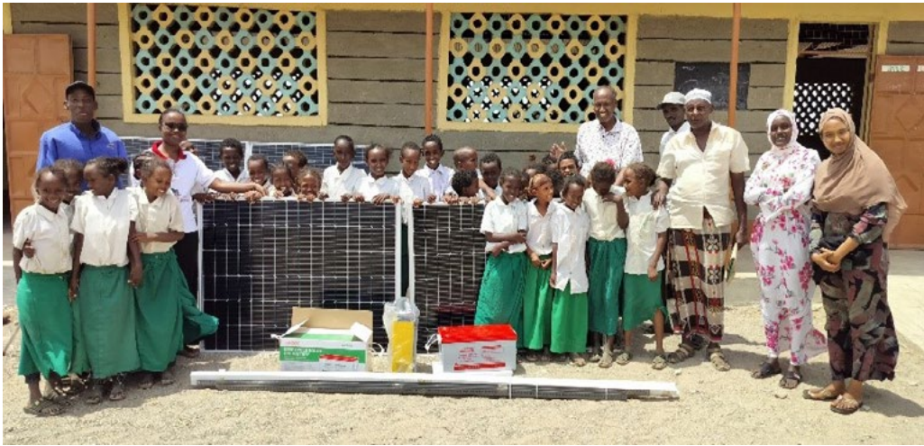
Shalom-SCCRR team: Ms. Esther Kibe MA, Habiba Dika BA, (MA Candidate) and Mr. Kennedy Oduor, delivering Solar System installation in one of the marginalized schools in Marsabit, northern Kenya. Shalom-SCCRR funded the Installation to provide lighting for both the pupils and the school administration.
